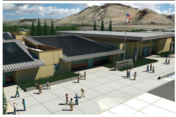
The new Romoland Middle School project demonstrates 2 important "green" strategies that were designed into the project. First, north-facing exterior walls are tall and generously fenestrated to take advantage of daylighting without introducing solar heat gains. Secondly, the sloped roof areas are south facing, making them ideal platforms for roof mounted photo voltaic panels for onsite renewable power generation. This project meets CHPS Design criteria.
